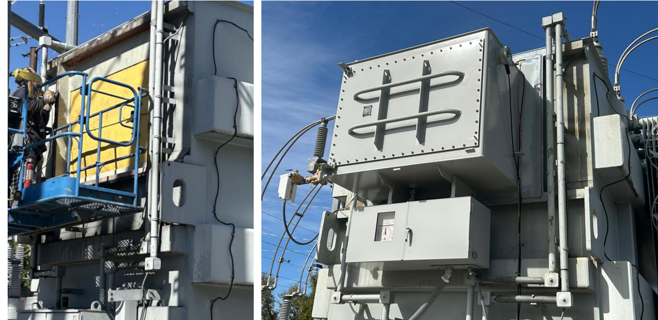
After LTC Replacement
