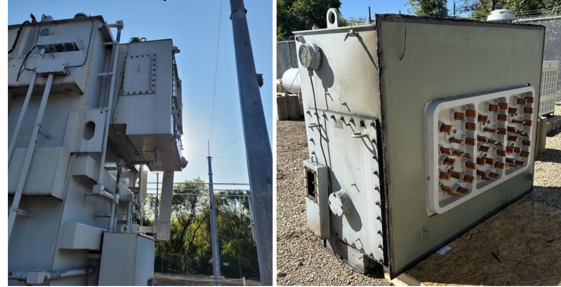
Before LTC Replacement
